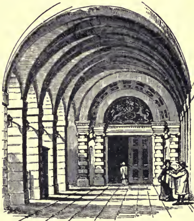
ENTRANCE DOOR, OLD COVENT GARDEN.
